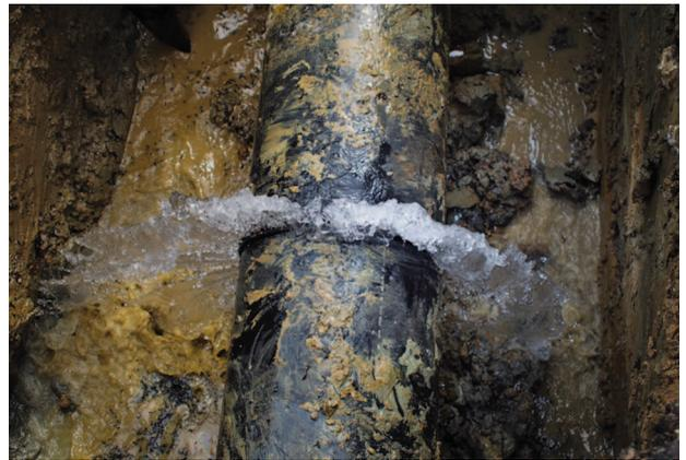
**Figure 5.** A leak in the legacy water supply infrastructure. (Image courtesy of Shutterstock.)
