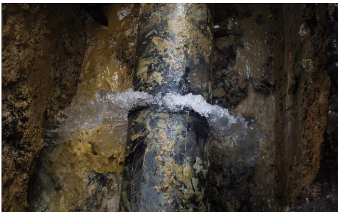
Fig. 5 Leak in the legacy water supply infrastructure
